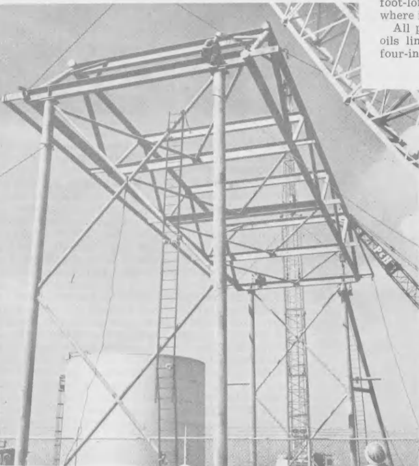
THE FOURTEEN-ton truss section of Lago's new pipe bridge was erected by the contractor March 19 with the aid of Lago's two heavy-duty cranes. Forty-foot columns support the section. E SECCION di aguante di diez-cuatro ton na e brug nobo di tubo na Lago a worde erigi door di e contratista Maart 19 cu ayudo di e dos gruanan pisá di Lago. Columnanan di cuarenta pia ta wanta e seccion.
